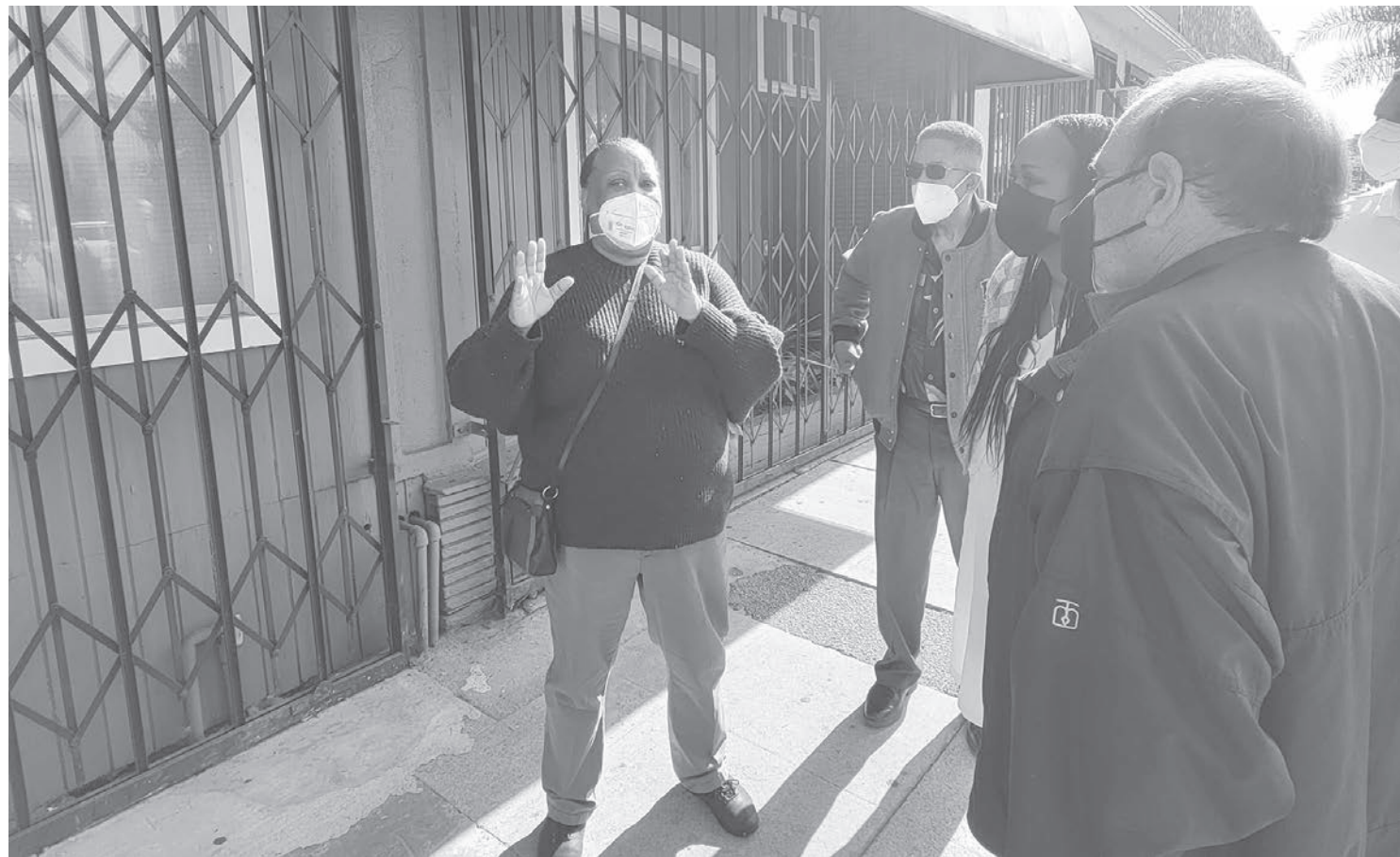
Al Wooten Jr. Youth Center Executive Director Naomi McSwain explains the required retrofits needed to reinforce the center from stray bullets. The after-school learning center has been hit by stray bullets at least five times since 2018. It recently received a $23,000 donation to cover the costs of installing bullet-resistant materials to the building's exterior.
